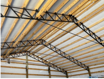
Gable Steel Trusses
