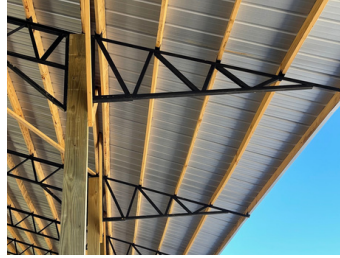
Snoot Steel Trusses
